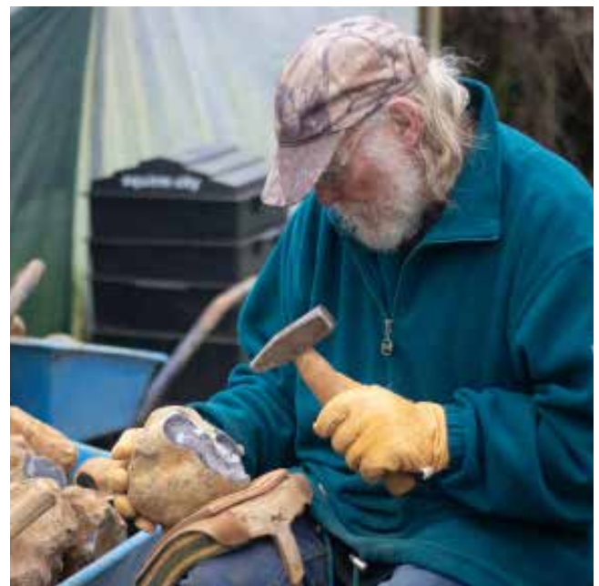
Flint knapping at St Mary's Church in Bungay, Suffolk, captured as part of the digital programme of technical training. (© CCT/George Reynolds)
