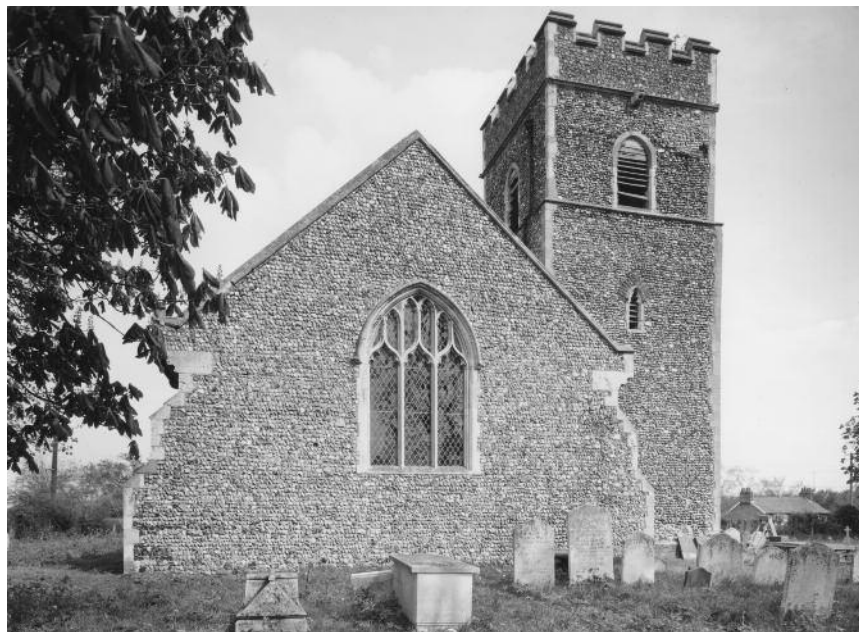
Exterior from the west (ROYAL COMMISSION ON THE HISTORICAL MONUMENTS OF ENGLAND)
