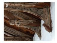
The nave has an impressive timber roof with alternating tie beams and false hammer beams. The tie beams have battlements across their length an on the gently curved supporting tir
