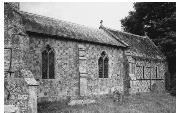
The chancel from the south
