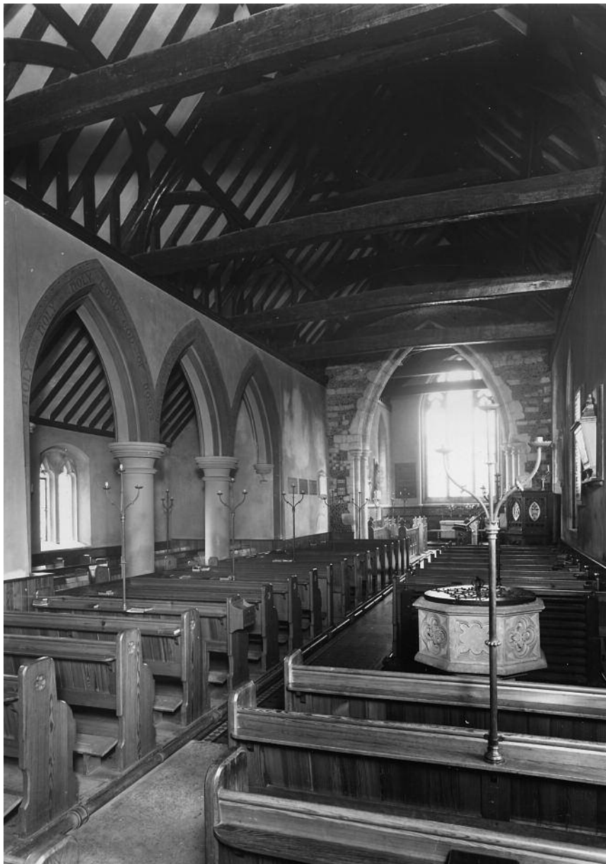
Interior looking east (ROYAL COMMISSION ON THE HISTORICAL MONUMENTS OF ENGLAND)
