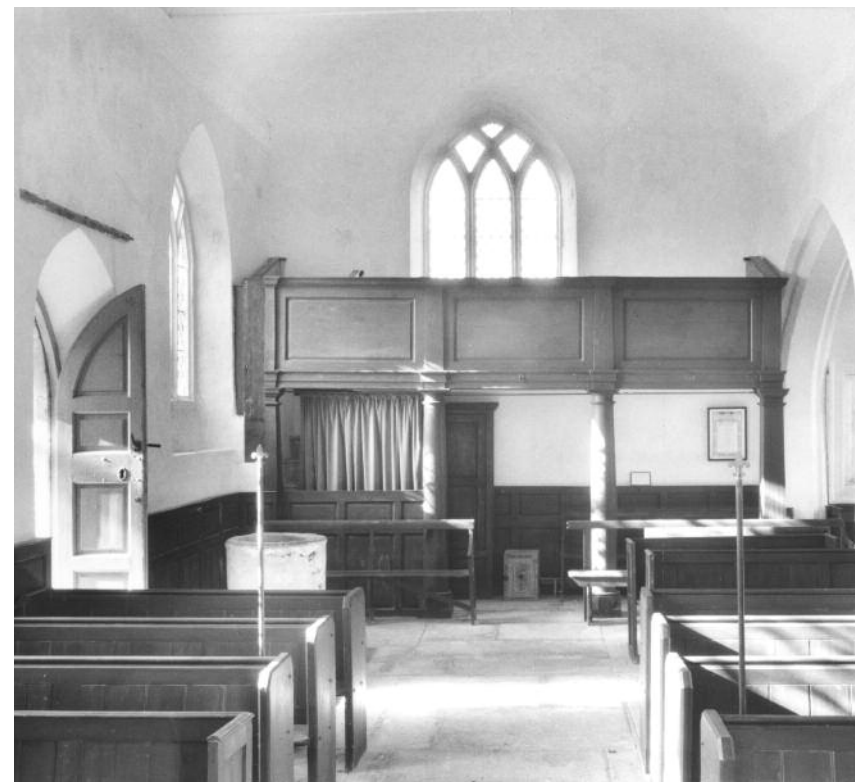
Nave looking west
