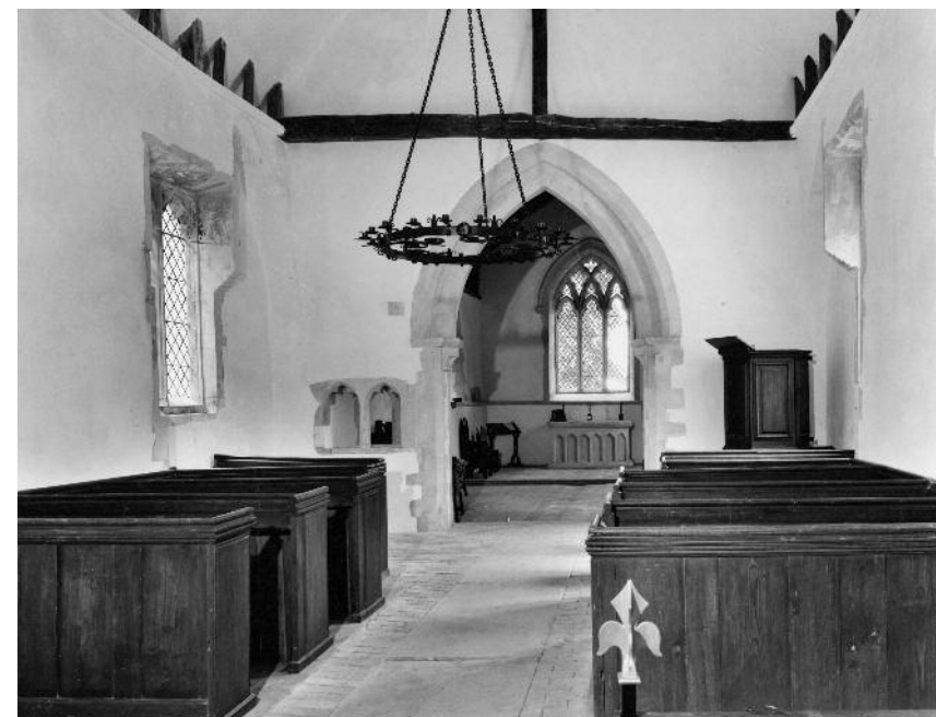
Interior looking eastwards
