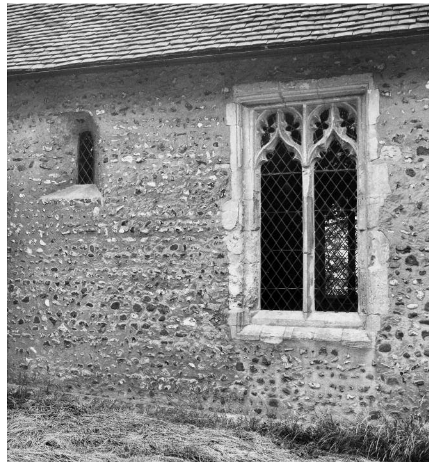
A thousand years of history in the south nave wall with its Saxon window and the larger window which was inserted 400 years later (CHRISTOPHER DALTON)
