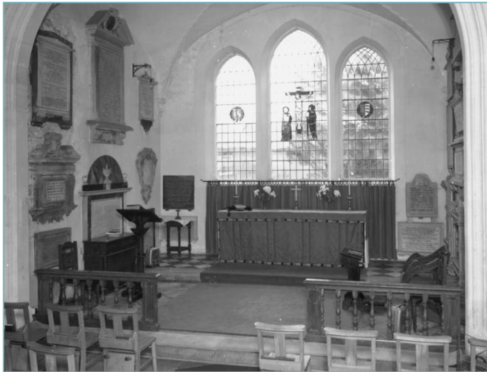
Interior from the south-west, with the chancel arch (© Crown copyright. NMR)
