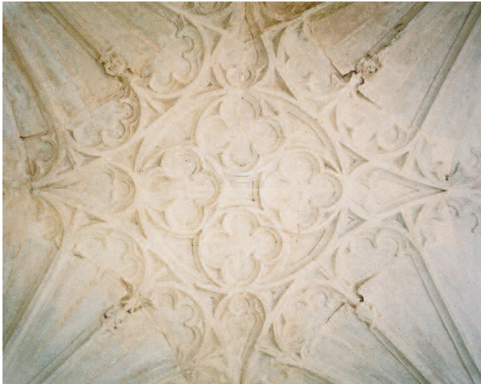
Vaulted ceiling in the south porch (Boris Baggs)
