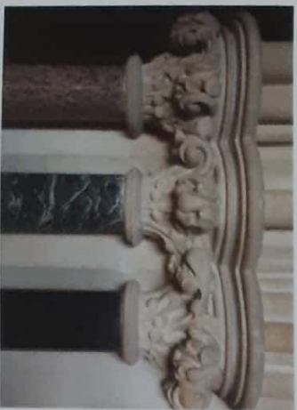
The ornate capitals and variegated stone shafts in the porch
