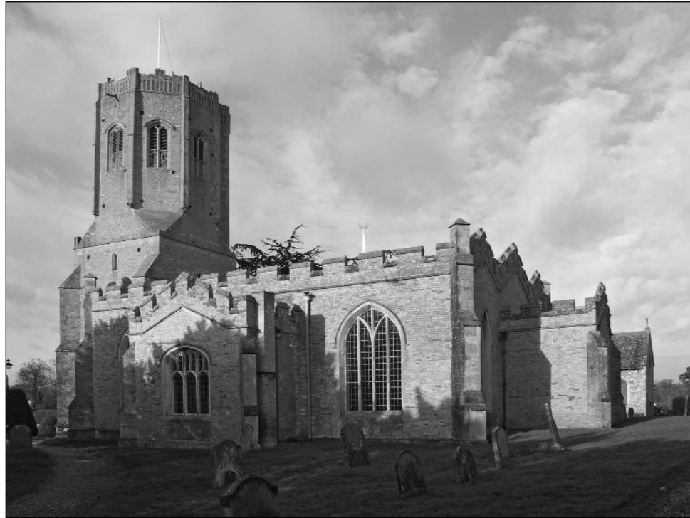
View from the south-west, showing both churches and churchyard
