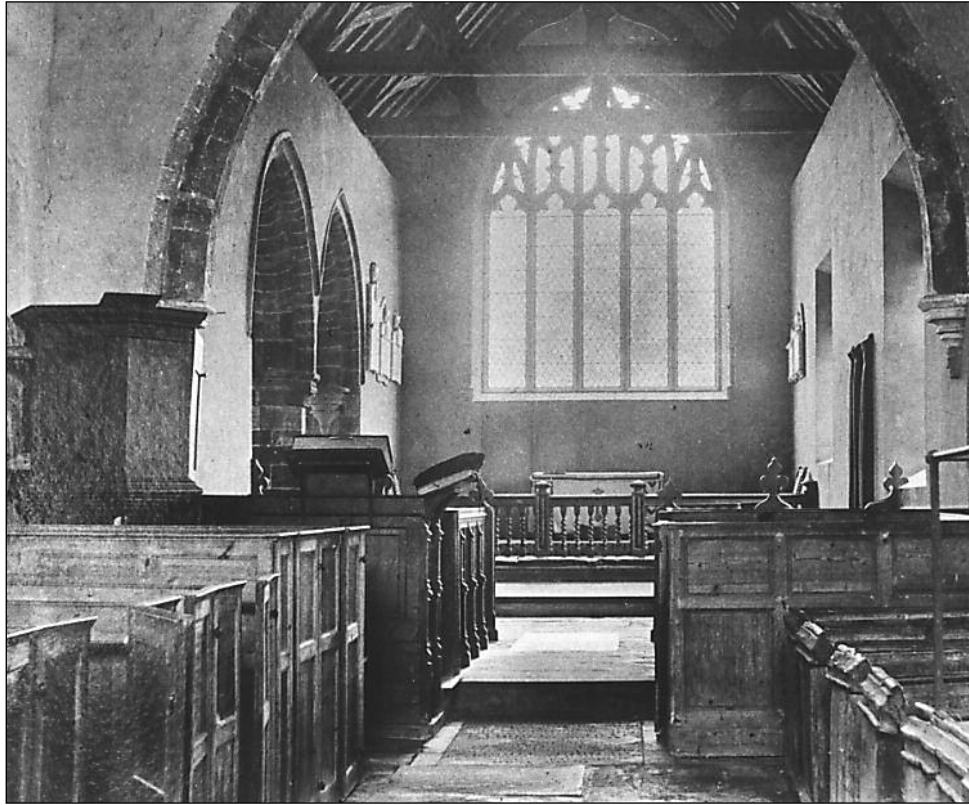
Before vandalism and repair.
