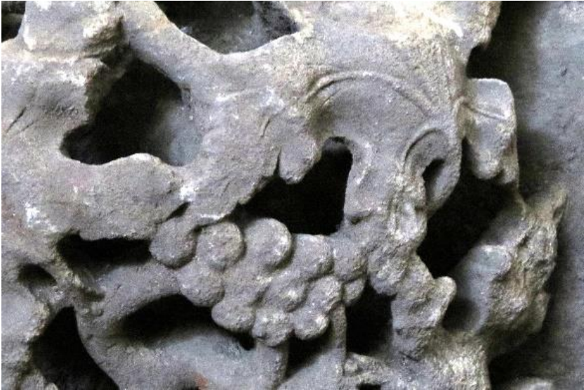
Above: Images of three of the St Thomas roof bosses.
